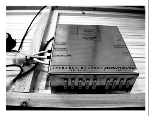
Connectingt Heater Cables: Plug the wires coming from the top of the wall panels into the color-coded Therapy (Yellow 5 total) and Celerant (Red 4 total) ports.
